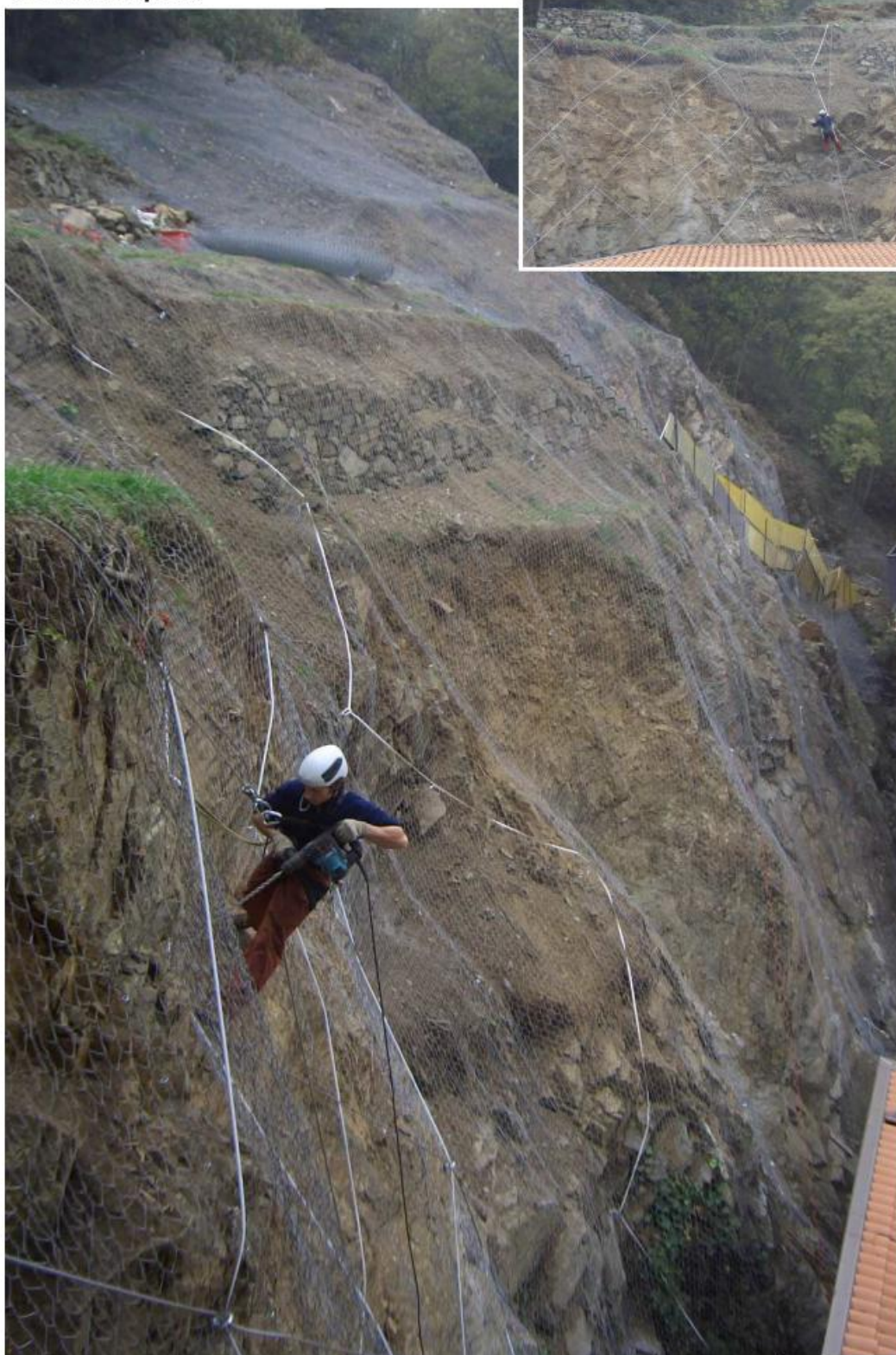
Messa in opera
